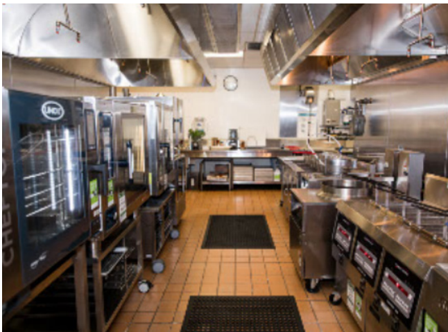
Commercially approved, installed and operational kitchen ventilation with commercial gas equipment properly installed beneath.
